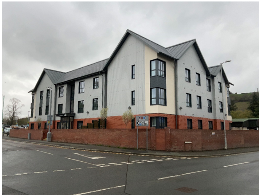
Newly built Council apartments in Newtown
